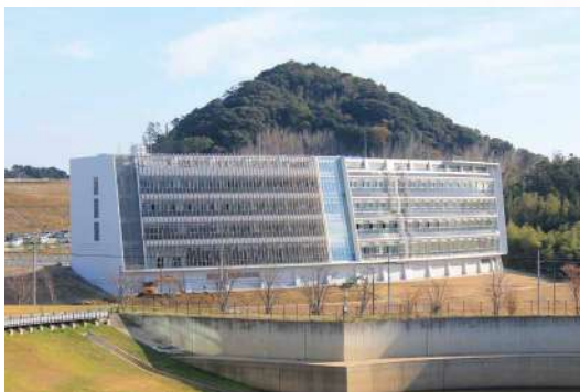
I 2 CNER Building circa 2013, during the early stage of Ito-campus consolidation
