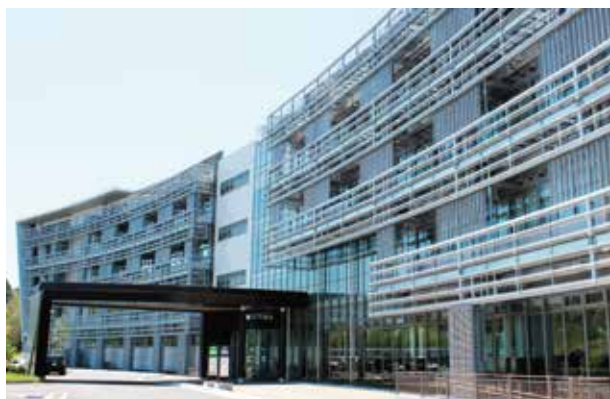
Main entrance of Building 1
